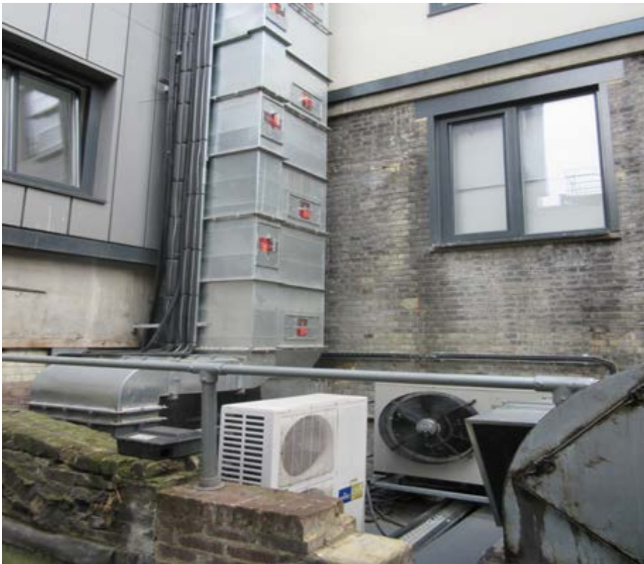
Photos to show installed extract ducts rising up the internal lightwell from 1 st floor level, adjacent bedroom windows of flats in 14 Bull Inn Court (metal clad part of the building).
